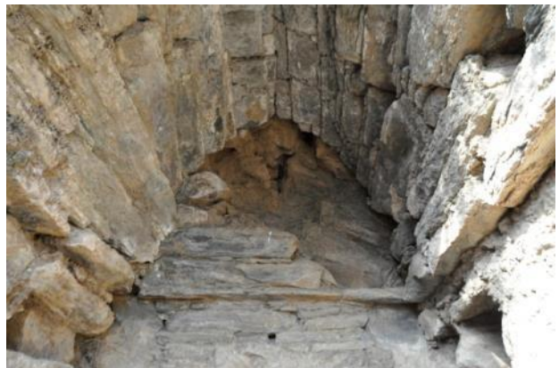
Plate-40. Corbelled roof at Kotona (Bampokha)
